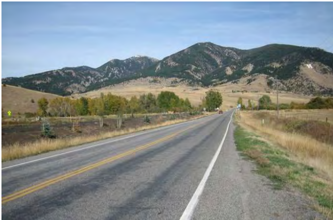
Photo 17: Bridger Drive has a variable shoulder along much of its length.
