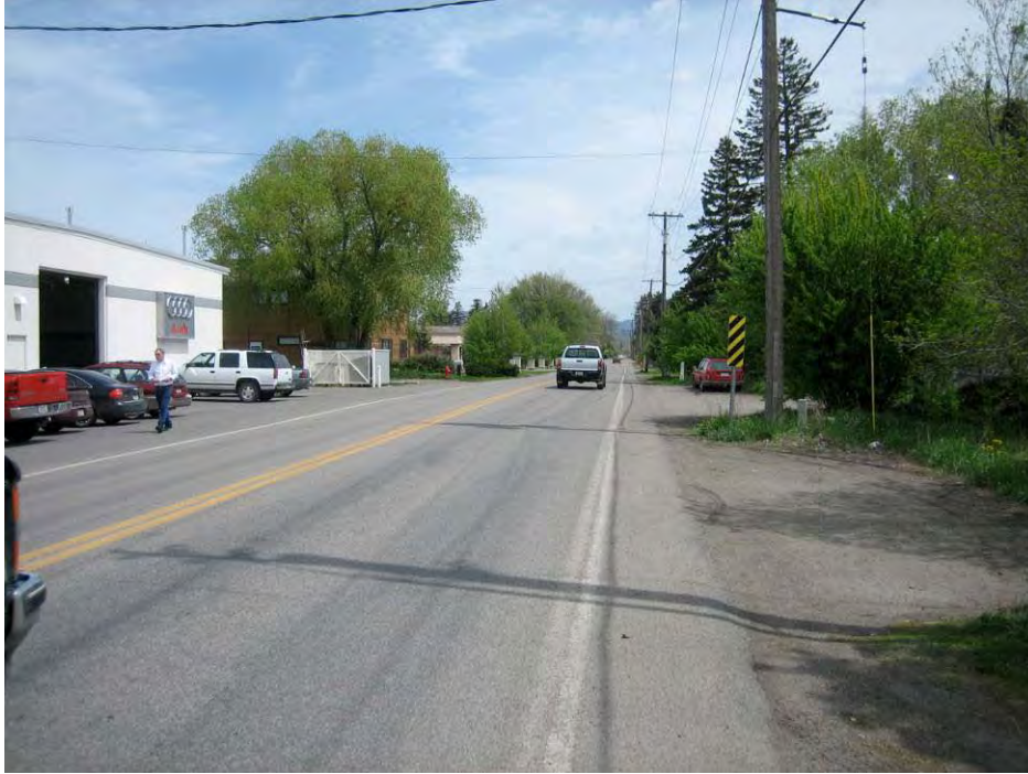
Photo 24: West Babcock Street (S. 19th to S. 11th Ave) acts as a major pedestrian corridor. Opportunities exist for expanded pedestrian facilities.
