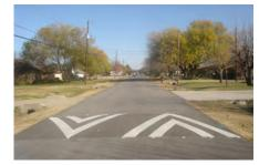
Speed humps are larger than speed bumps and range from 3 to 4 inches high and 10 to 14 feet long. They can be used on streets where a low speed limit is desired. Speed humps generally can slow vehicles down to approximately 15 miles per hour. If traveled over at higher speeds the vehicle will experience a severe jolting effect.
