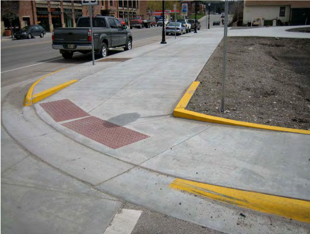
Photo 3: Newly reconstructed sidewalks in downtown Bozeman have ADA-compliant ramps.
