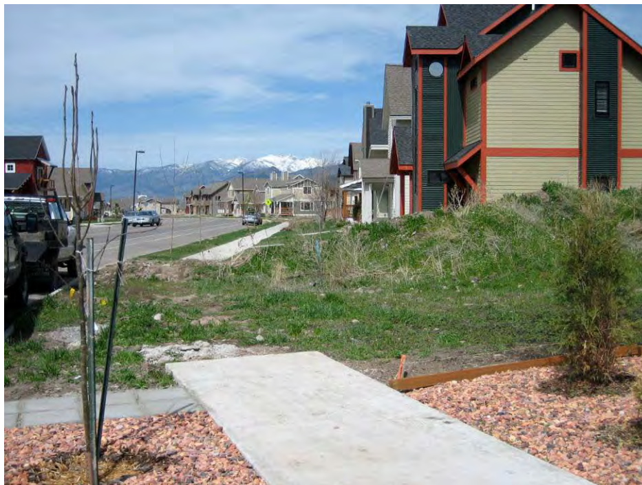
Photo 23: Sidewalk gaps in new development areas can exist for up to 3 years. At the end of 3 years the developer is required to finish any undeveloped sidewalk sections.
