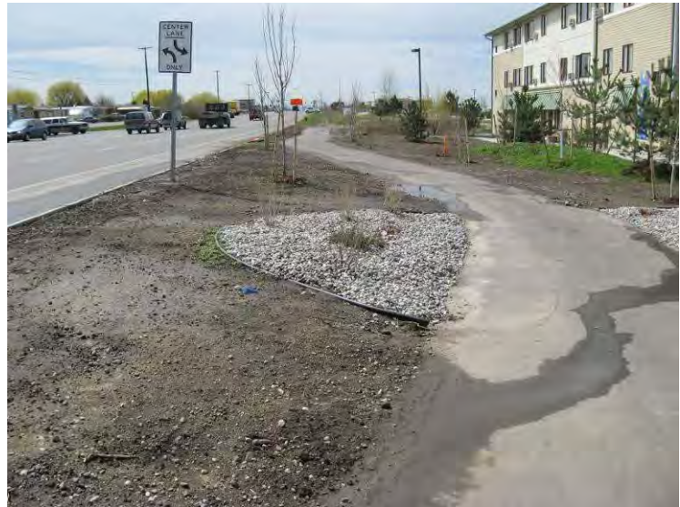
Photo 20: A shared-use path has been installed on Oak Street.
