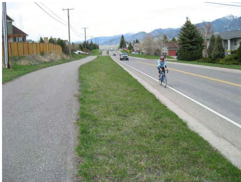
Photo 5: This cyclist chooses to ride along the shoulder of Highland Blvd. rather than on the adjacent shared use path.
