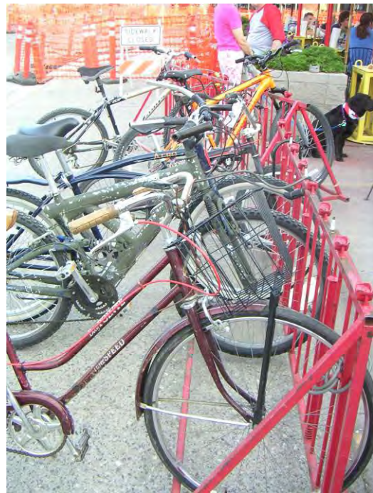
Photo 15: These outdated “comb” type bike racks at a local restaurant are considered a less desirable rack design because it is difficult to lock the frame to the rack.
