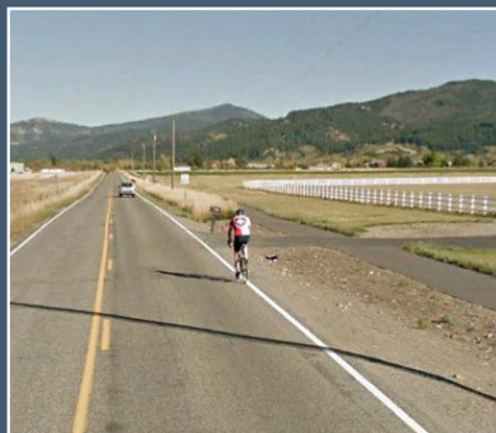
Rural roadways, such as South 19th Avenue pictured above, typically include paved shoulders instead of curb and gutter and rely on on-street bicycle facilities or separated paths for non-motorized use.
