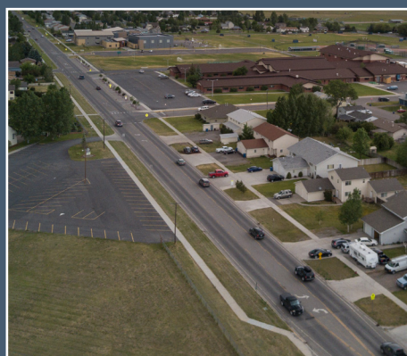
Urban roadways, like Jackrabbit Lane within the Belgrade Urban Area, typically include curb and gutter, bike lanes or bike boulevards, and sidewalks often separated by grassy boulevards.
