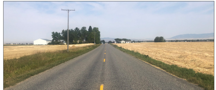
Road design standards help provide a uniform and predictable driving environment and help provide safe accommodations.
